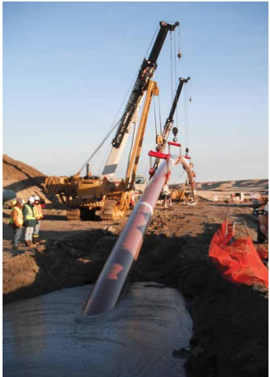
*Proper alignment with the drilled hole is critical for safe installation*
